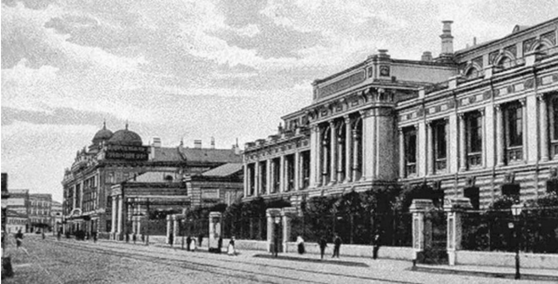
The State Bank of the Russian Empire in 12 Neglinnaya Street, Moscow. This same building now houses the The Central Bank of the Russian Federation.
